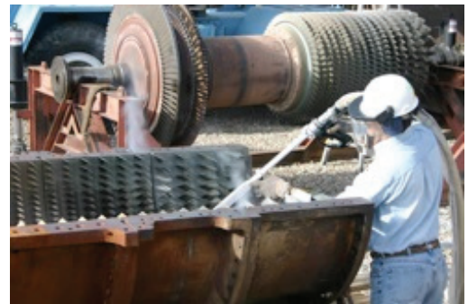
Cleaning a turbine at Rifle Generating Station. Combustion residues are blasted loose with dry ice.
