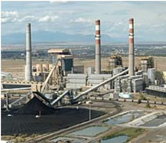
Comanche Generating Station, near Pueblo At 1426 MW, the largest power plant in Colorado Burns Wyoming coal in 3 units Operated by Xcel Energy
