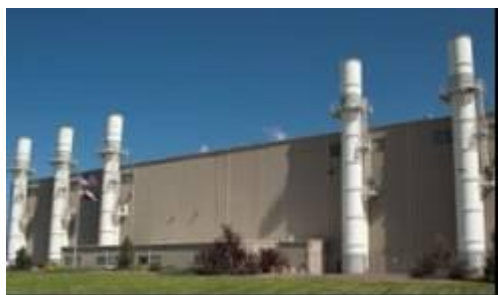
J. M. Shafer Generating Station in Fort Lupton Natural gas fuel. Combined cycle operation. 272 MW from 5 units. Owned by Tri-State.
