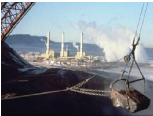
View of Craig Station from Trapper Mine
